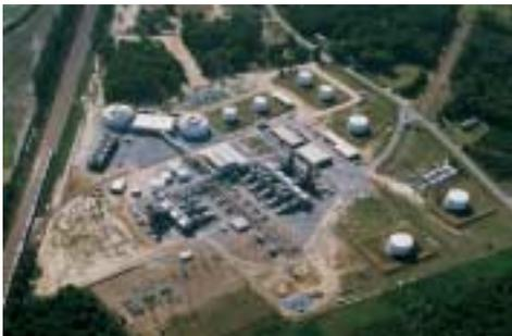
The **Butler-Warner Power Plant** in North Carolina – the world's largest thermal energy storage (TES) project to date – depends on a half-a-million feet of stainless steel tubing in 112 Heatcraft custom coils to help cool air used in generating electricity. The 112 cleanable Heatcraft coils were custom-made, delivered and installed one week ahead of schedule.
